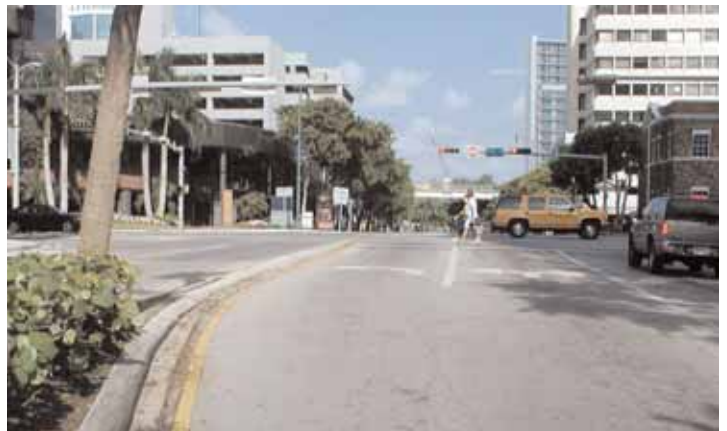
This left turn lane on SE 8th Street heading west will be lengthened to enable more storage.
