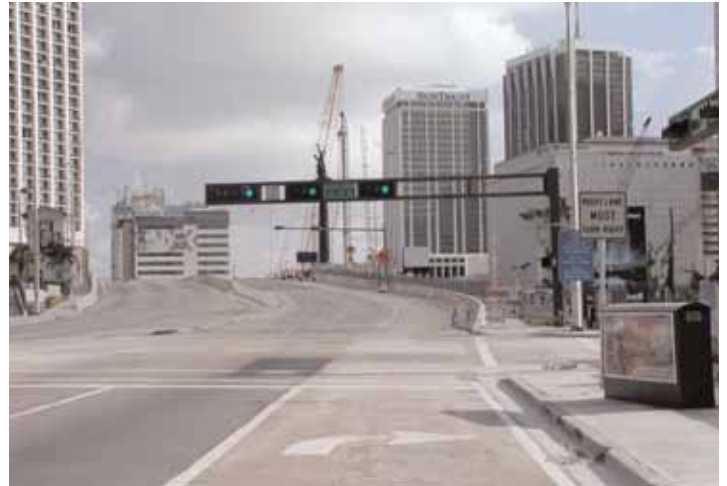
Additional northbound lane over the Brickell Bridge under construction.
